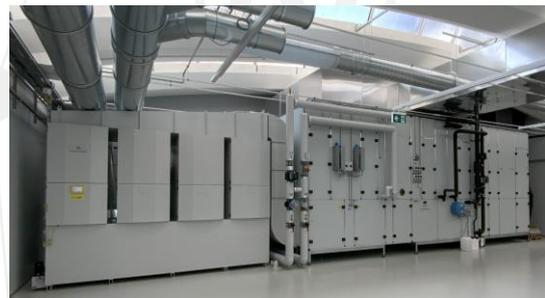
Figure 4: Oil smoke filter connected to the central ventilation unit
