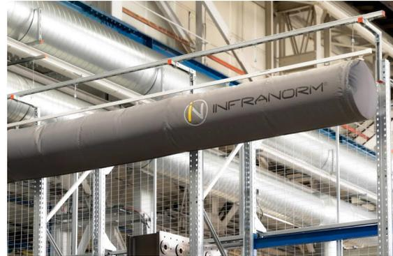
Figure 5: The textile air outlets for the draught-free supply of cooled fresh air.
