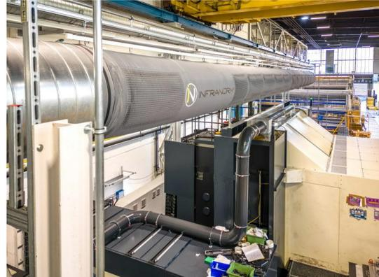
Figure 9: Workplaces are supplied with pleasantly cool fresh air by means of an adiabatic cooling system.
