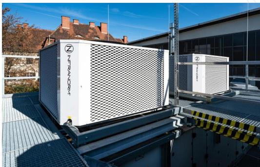
Figure 3: Mixed air unit with top-mounted two-stage adiabatic cooling for 28.000 m³/h
