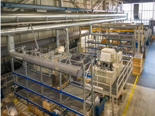
Figure 8: The air is introduced target-oriented in zones with the individually manufactured textile air outlets.
