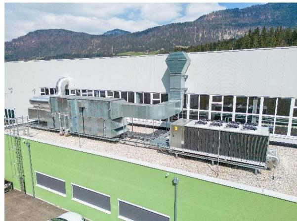
Figure 3: Supply and exhaust air system for machine halls and reversible heat pump
