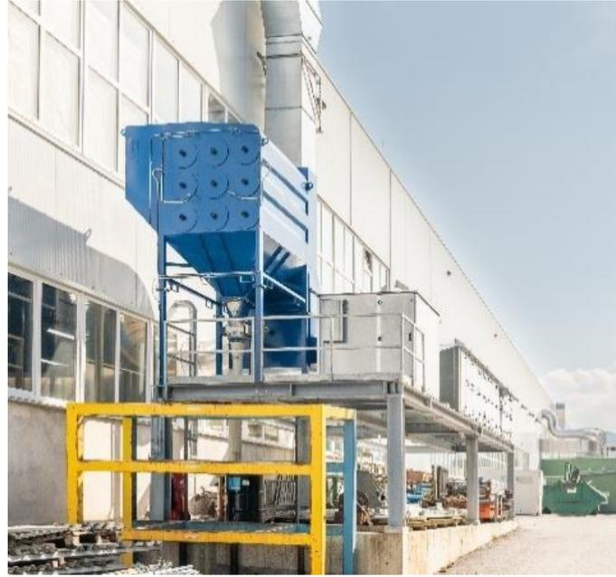
Figure 9: Cartridge filter with exhaust air unit and (in the background) ventilation unit - grinding shop area
