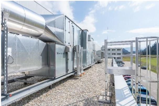
Figure 6: Ventilation system with rotary heat exchanger - machine hall area
