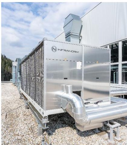
Figure 10: Reversible heat pump for heating and cooling the entire site in Grub
