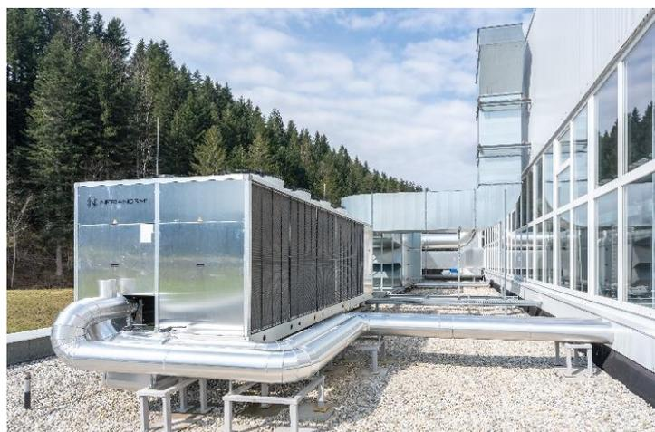
Figure 11: The reversible heat pump is mainly powered by the new photovoltaic system at the Grub site
