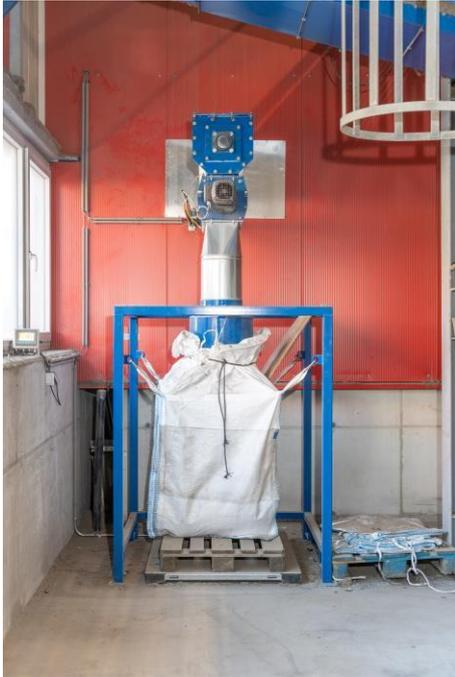
Figure 9: Pressure-decoupled dust discharge with electronic weighing unit
