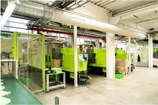
Figure 8: The air is introduced in a focused manner for the employees with the individually manufactured textile air hoses.
