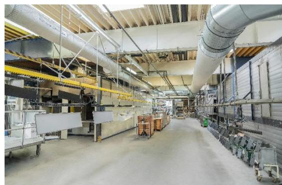
Figure 5: The textile air hoses for the draft-free supply of cooled fresh air.
