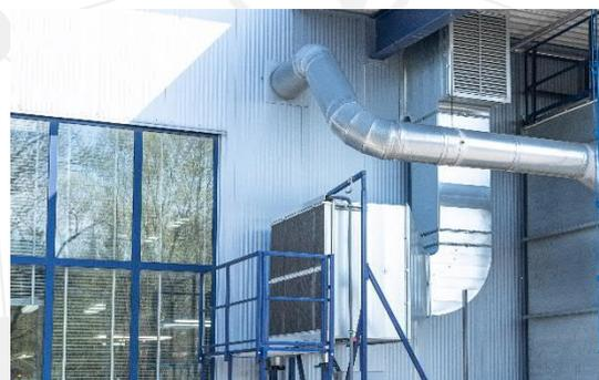
Figure 4: Single-stage adiabatic pre-cooling of the intake air of the existing ventilation unit
