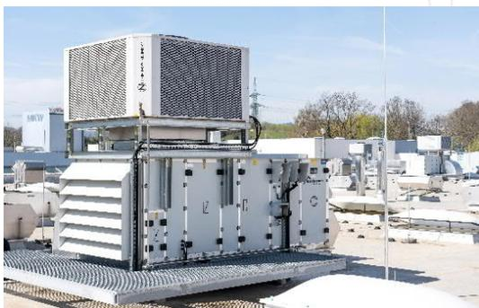
Figure 3: Mixed air unit with top-mounted two-stage adiabatic cooling system
