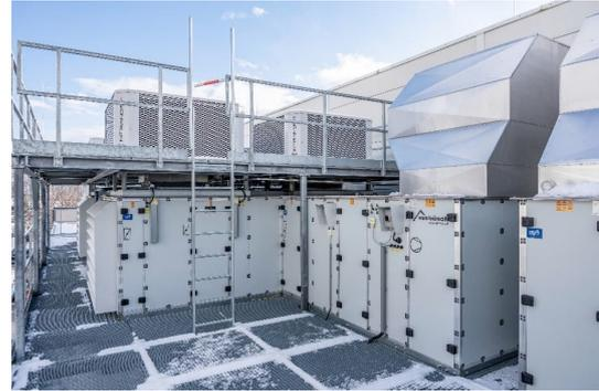
Figure 9: Ventilation units with attached cooling units for year-round air conditioning.
