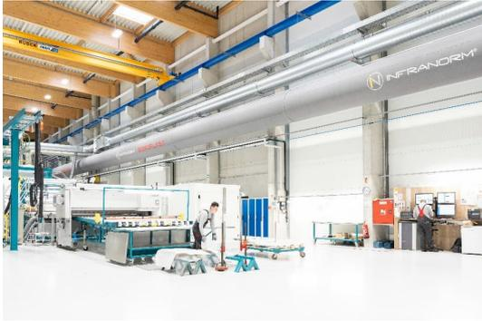
Figure 8: The air is introduced with the individually manufactured textile air outlets.
