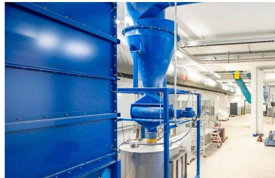
Figure 5: The mill cellar operated with negative pressure for recycling the production waste.
