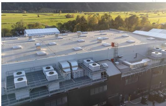
Figure 3: Exterior view of the plant for up to 126,000 m³/h cooled fresh air supply
