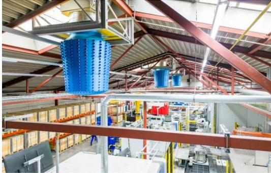
Figure 6: Space-saving installation in the existing strip lighting
