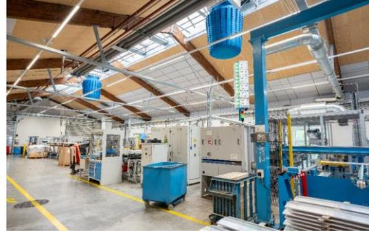
Figure 7: Air supply with textile air outlets without the need for piping
