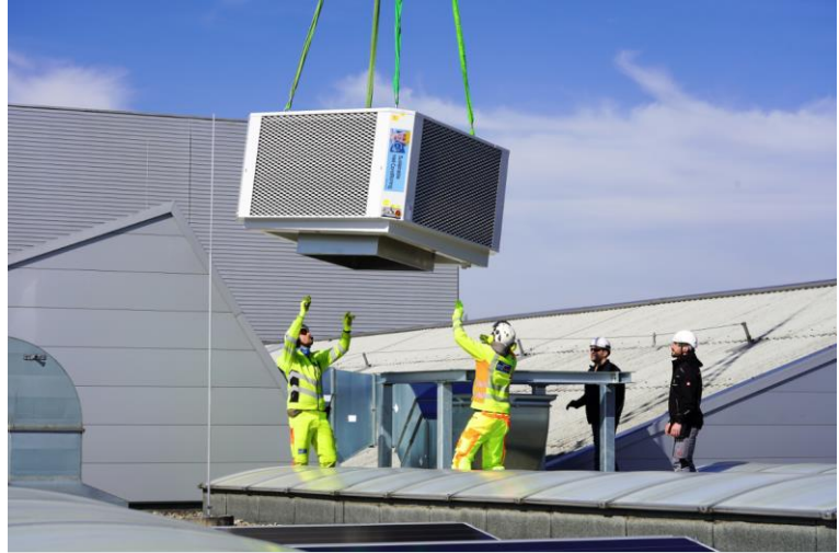
Helicopter transport of elements to centrally located hall.
