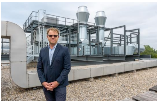
Figure 3: Technical Director DI Gerhard Typelt in front of the new plant
