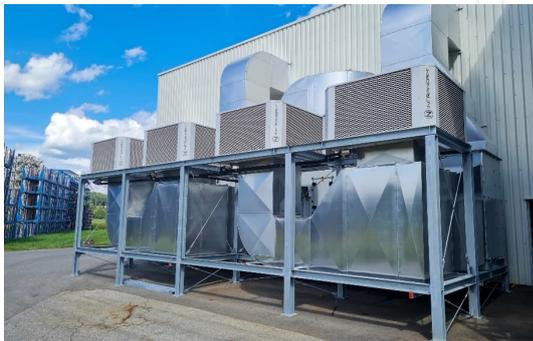
Figure 3: Installation of the adiabatic cooling units next to the ventilation units
