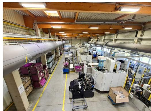
Figure 5: The textile air hoses for the draught-free supply of cooled fresh air.
