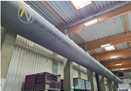
Figure 6: Textile air outlet with laser perforation
