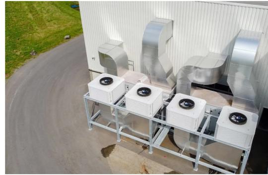
Figure 9: Two-stage adiabatic cooling units with air handling units and ductwork
