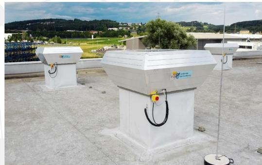
Figure 4: Roof fans for heat removal from the hall and pressure control
