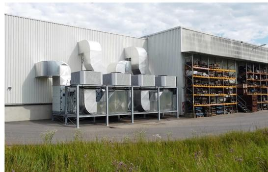
Figure 7: Installation of the adiabatic cooling units in the outdoor area
