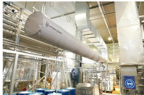
Figure 5: The textile air hose for the draft-free supply of the cooled fresh air.
