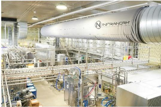
Figure 6: In cooling zones, textile air hoses introduce the pleasantly cool fresh air.
