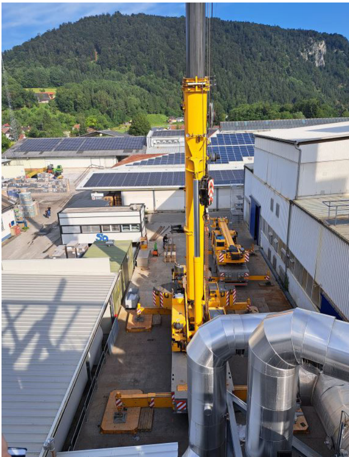
Image 03 and image 04: Two cranes were used for the work: one took over the precise lifting of the heat exchanger, while the other was used for assembly work with a crane cage.
