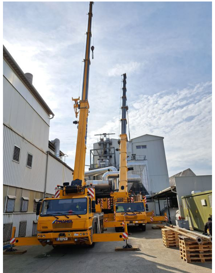
Image 03 and image 04: Two cranes were used for the work: one took over the precise lifting of the heat exchanger, while the other was used for assembly work with a crane cage.
