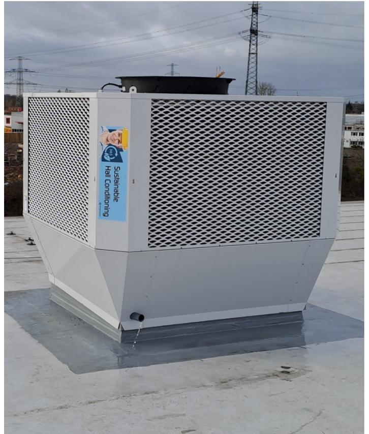
**Image 03:** The two-stage IntraCool adiabatic cooler uses natural evaporation cooling to efficiently reduce temperature and minimize energy consumption.
