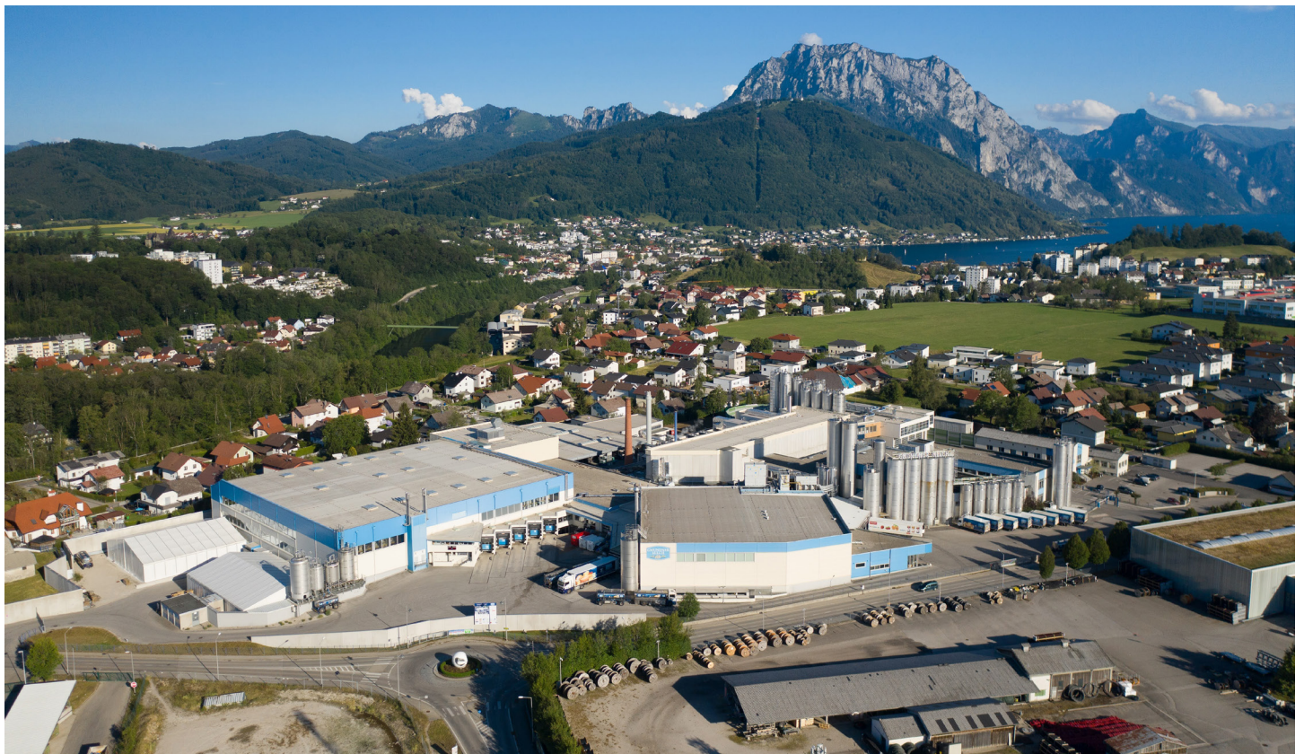
Image 01: Modern and efficient production facilities ensure that customers can produce high-quality dairy and cheese specialties in a cost-effective manner.
