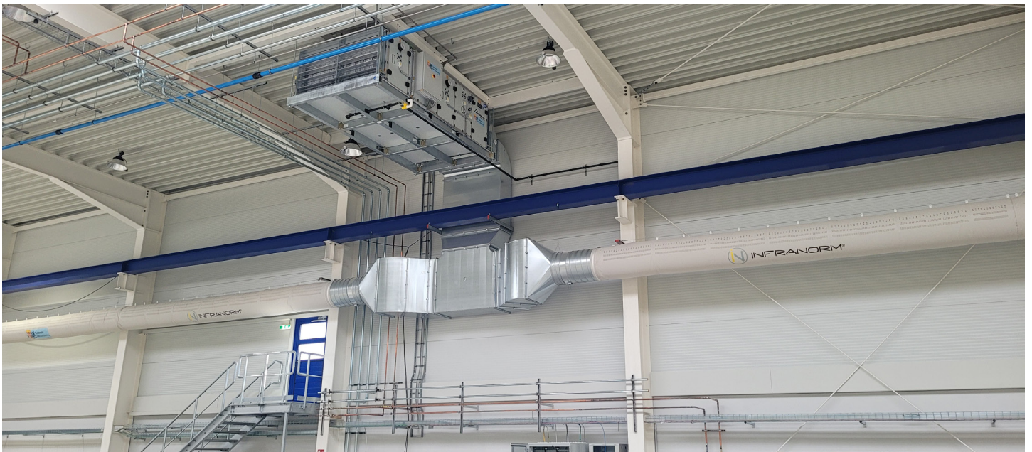
Image 04: The textile supply air hose system ensures a draft-free and even distribution of the conditioned air.
