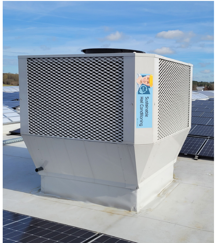
Image 03: The two-stage IntrCooll adiabatic cooler uses natural evaporation cooling to efficiently reduce temperature and minimize energy consumption.
