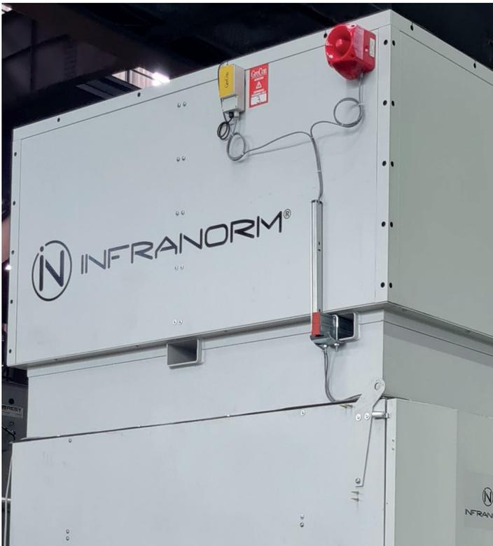
**Image 03:** Cost-effective filter system with spark detector and signal horn for early fire detection
