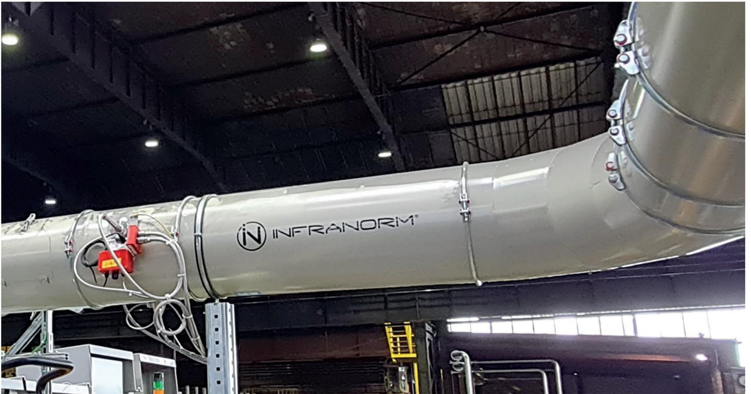
**Image 02:** Innovative extraction system with spark detector for early fire detection
