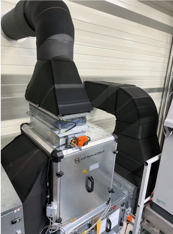
Picture 03: Detailed view of the INFRANORM® heat recovery unit in stainless steel design – compact, easy to maintain, and designed for maximum durability.
