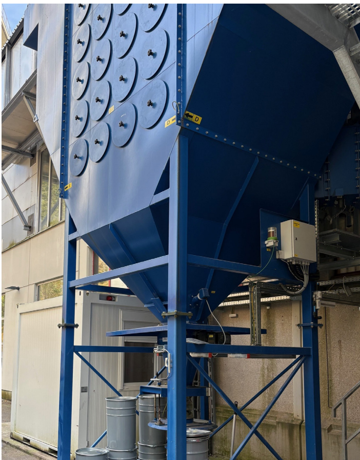
Image 06: Filter system and barrel container for the application of filtrate (Project 2)
