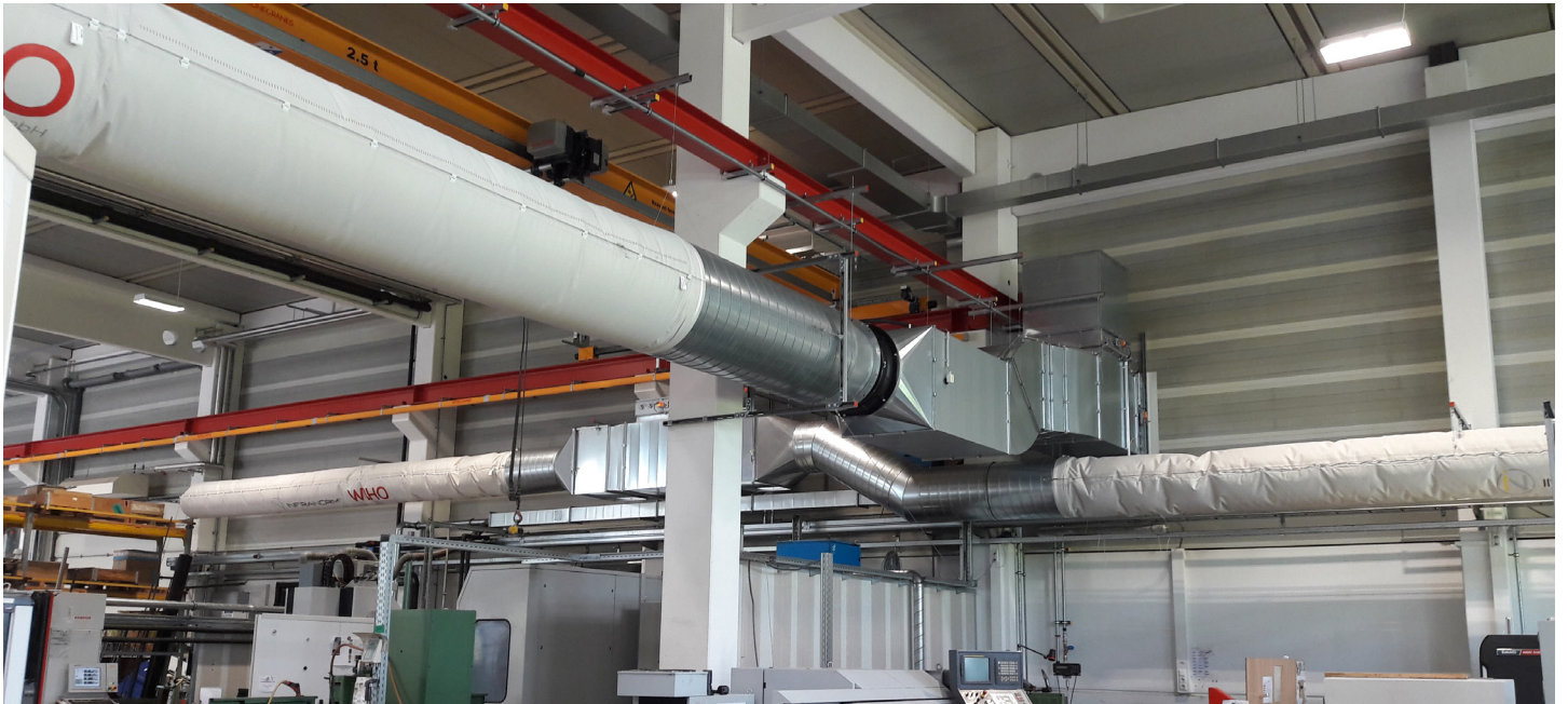
Image 03: Airflow management and system integration in the production area for targeted temperature control and stabilization of indoor conditions
