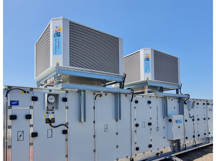
Image 03: Modular indoor air conditioning system with adiabatic cooling and integrated system technology
