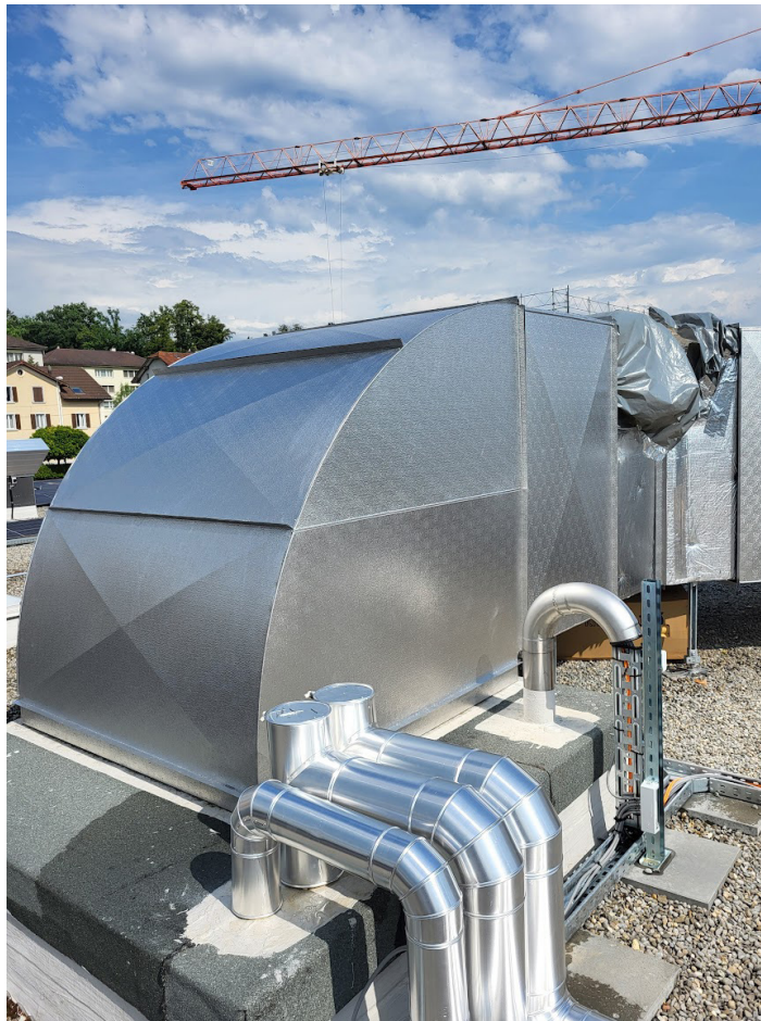
Image 01: Installation of the indoor air conditioning system using a crane while operations continue
