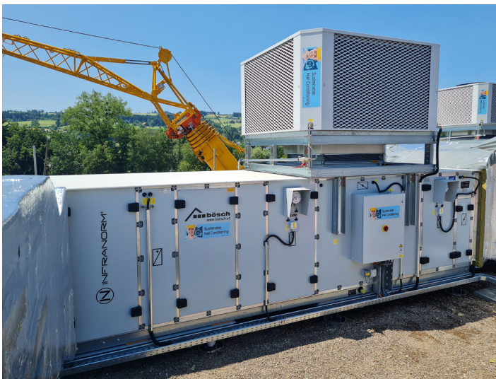
Image 04: Installation of the indoor air conditioning system in accordance with project-specific requirements
