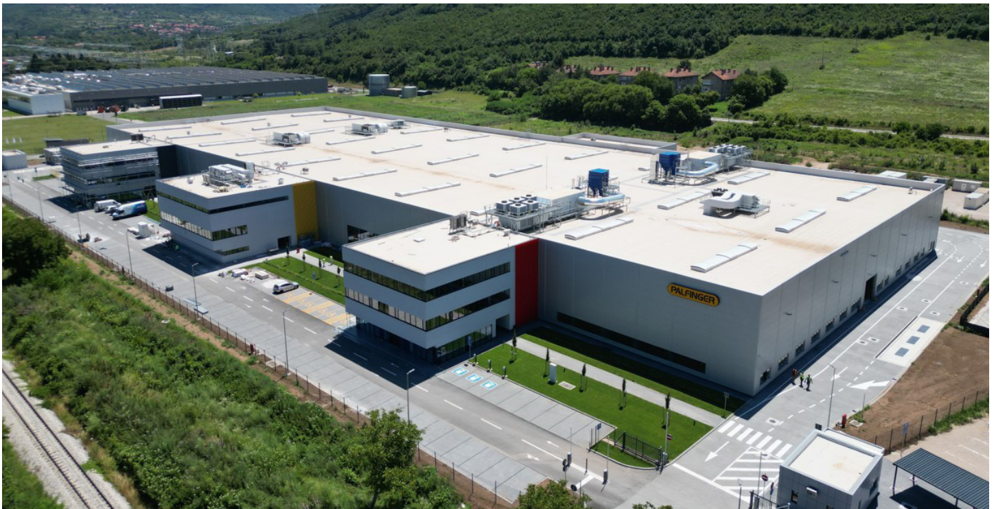
Image 03: Construction of the new PALFINGER production facility in Niš, featuring integrated infrastructure for indoor climate control and air purification
