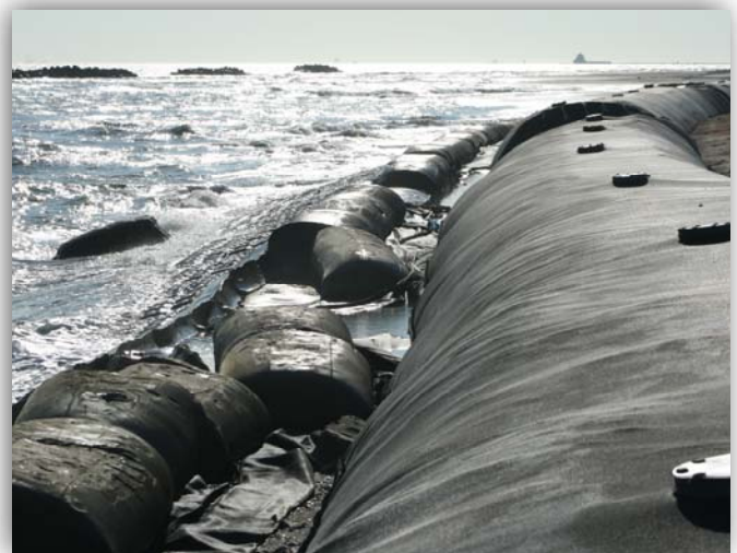
FIGURE 9 — Boudin Bags in Front of GeoTubes November 2, 2017
