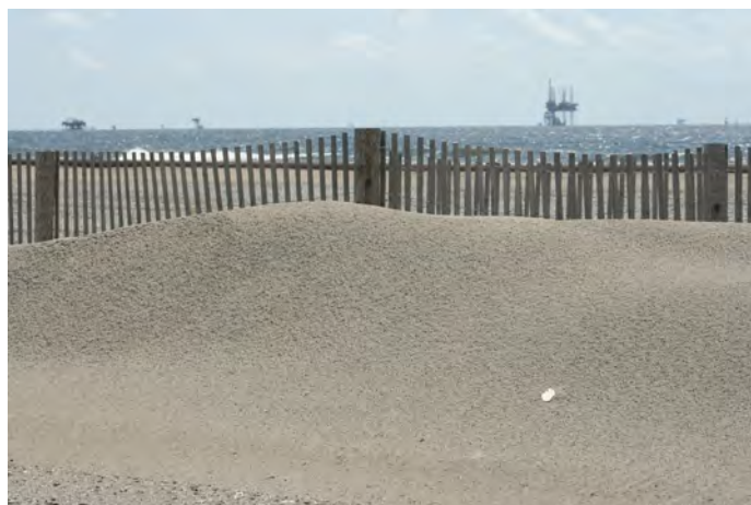
FIGURE 57 — Sand Fencing on CAM I Area September 4, 2014 Photo Courtesy of L. Amanda Phillips
