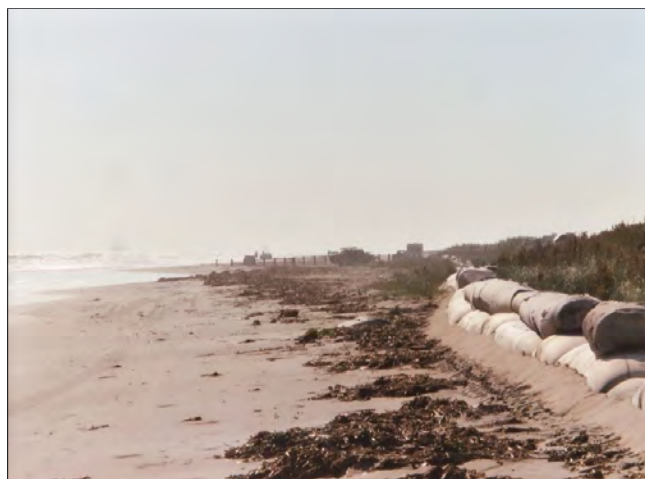
FIGURE 4 — Boudin Bags at the Foot of Highway 3090, Fourchon, Lafourche Parish November 1, 2003
