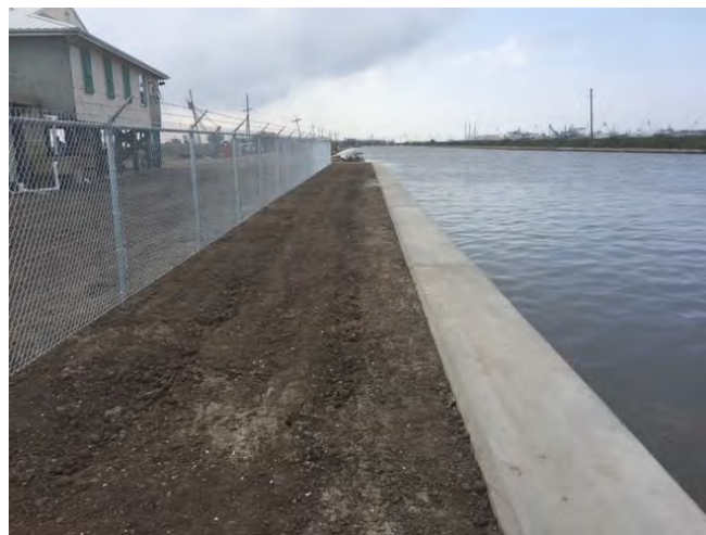
FIGURE 32 — LUMCON Repaired Bulkhead Lafourche Parish March 29, 2016
