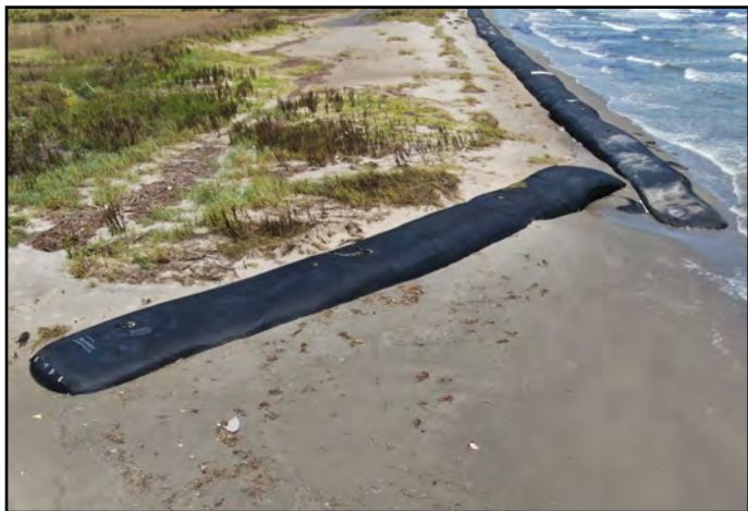
Western end of GeoTubes post-Barry - Fourchon Island, Lafourche Parish. July 16, 2019. Courtesy of Comeaux Consulting Group.
