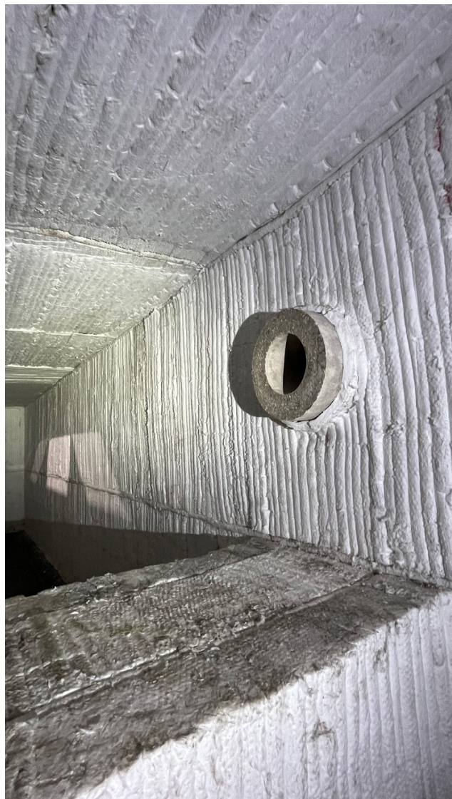
Fig. 3 The H-Anchor System allows for flexibility of anchor placement to accommodate lining penetrations such as burner blocks.
