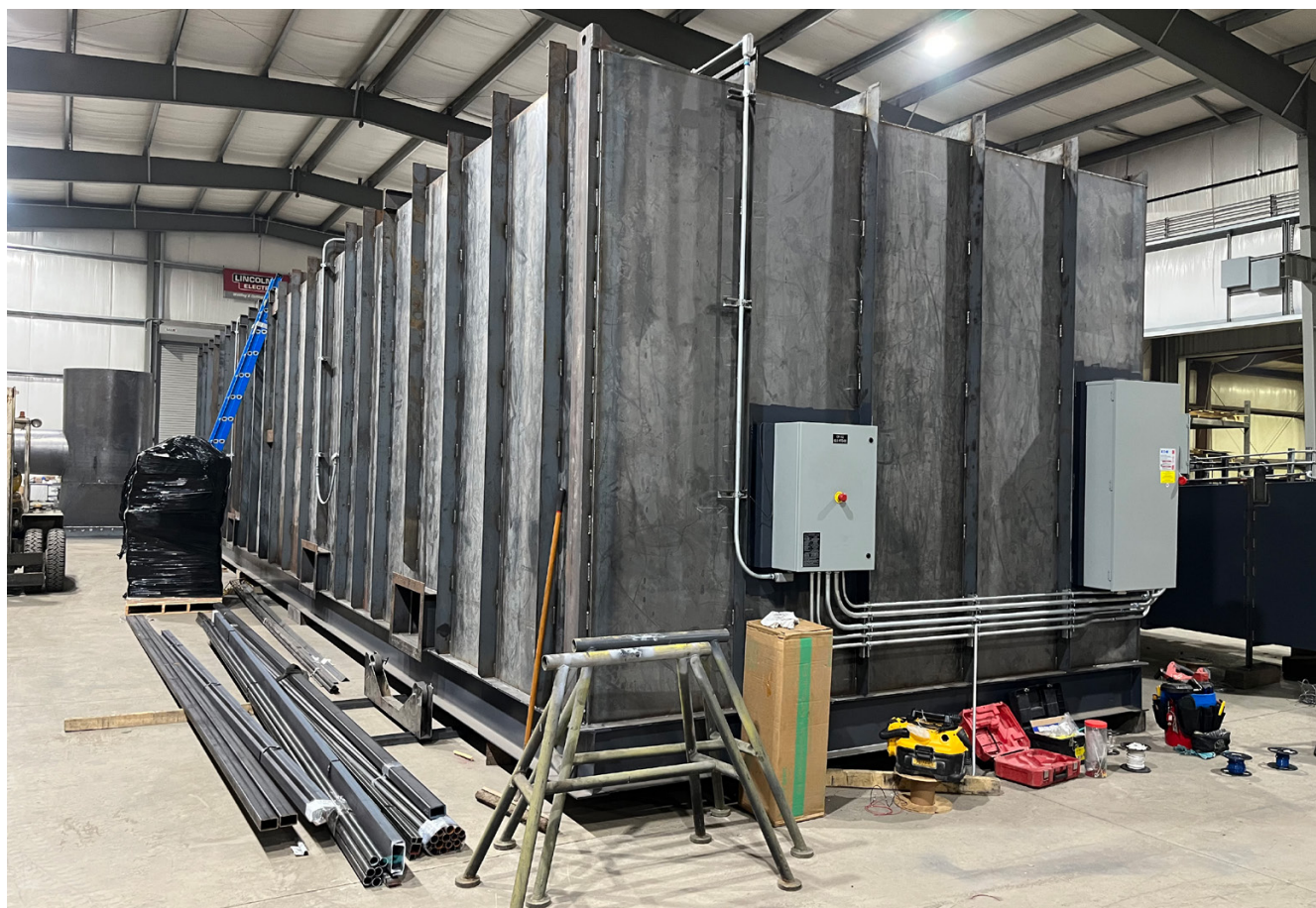
Fig. 1 Typically, fiber installation takes place at the steel fabrication facility. MaxBlock modules provide a light weight insulation system which can be installed using unskilled labor.
