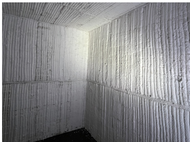
Fig.6 Since they are larger than most typical modules, MaxBlock modules in conjunction with the H-Anchor System install quickly and minimize seams throughout the insulation system.
