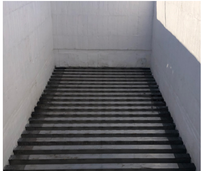
Fig.3 Typical Regenerative Chamber Section
