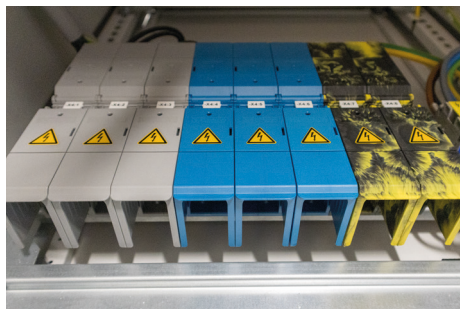
Phoenix RBO Connectors for DUT Connections
