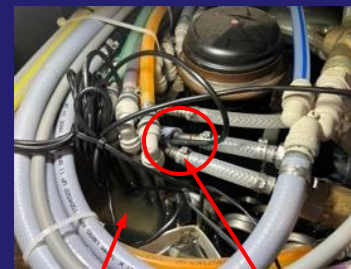
Temperature probe – Water Flow to Drinks Tower
