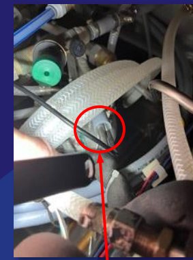
Temperature probe – Return Flow from Drinks Tower
