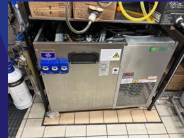
Multiplex 44 Icecore Cooler/Carbonator
