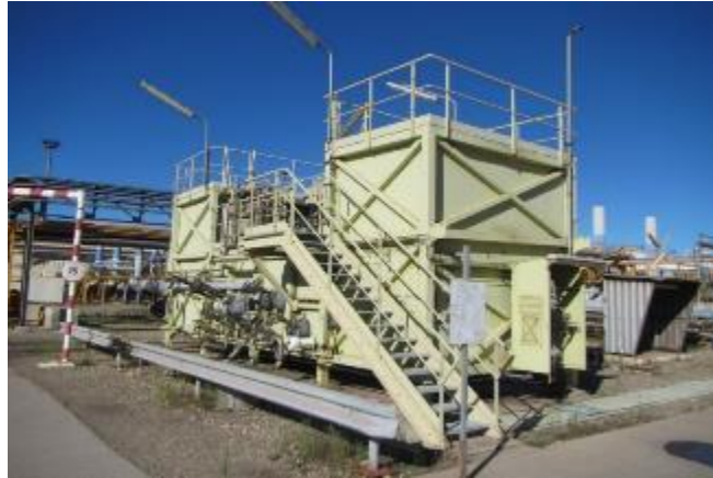
Figure 13. Picture of N2/ LNG heat exchanger at Fos Tonkin terminal
