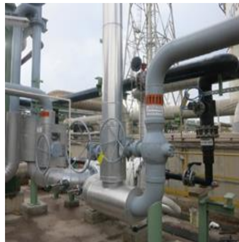
Figure 26. BOG/sea water heat exchanger
