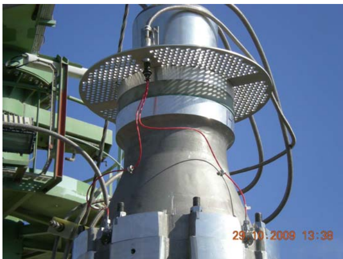
Figure 5.- Accelerometer directly attached to the LNG pump (an in-tank pump in this case). Accelerometer in contact with LNG.
