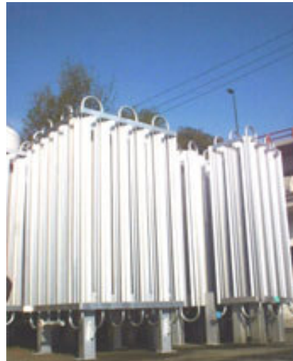
Typical ambient air liquid nitrogen vaporisers
