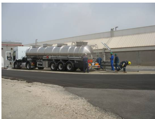
Impounding area for truck unloading
