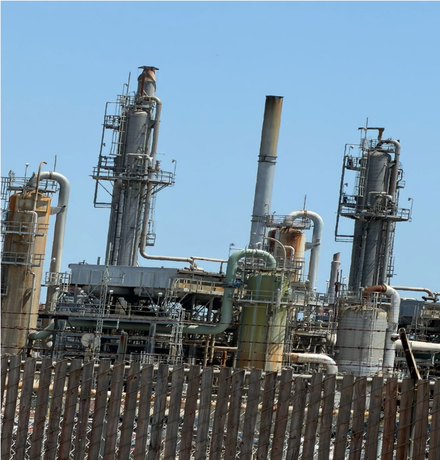
The Phillips 66 refinery in Carson has been operating for over 100 years. Carson residents are pushing for a remediation plan that benefits communities rather than continues the legacy of harm. (Photo by K Sanchez)
