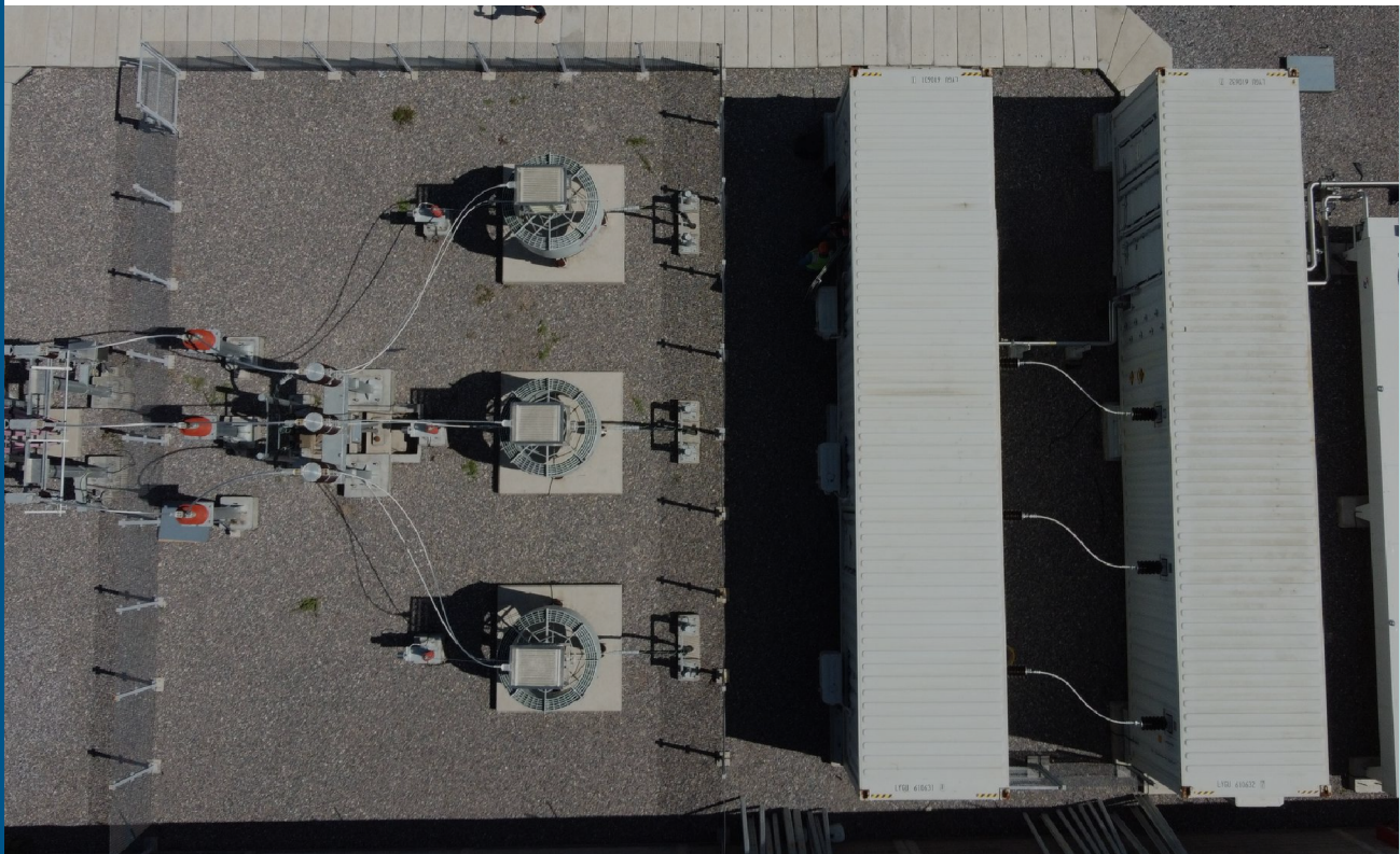
Figure 4. Upgrading 80 Mvar SVC with 40 Mvar STATCOM
