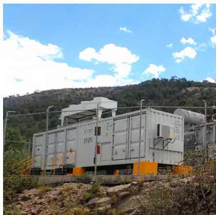
Mining 6 MVAR STATCOM
