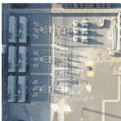
Steel (EAF) 320 MVAR STATCOM
