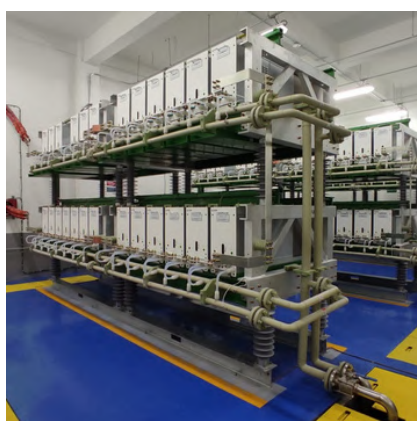
Steel (EAF) 120 MVAR STATCOM
