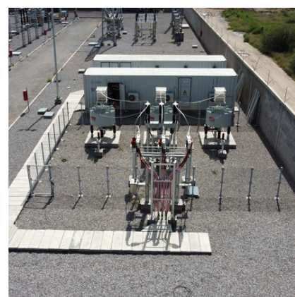
Steel (EAF) 40 MVAR STATCOM
