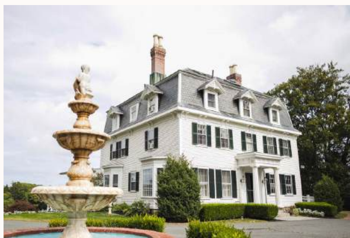
THE ESTATE HOUSE
