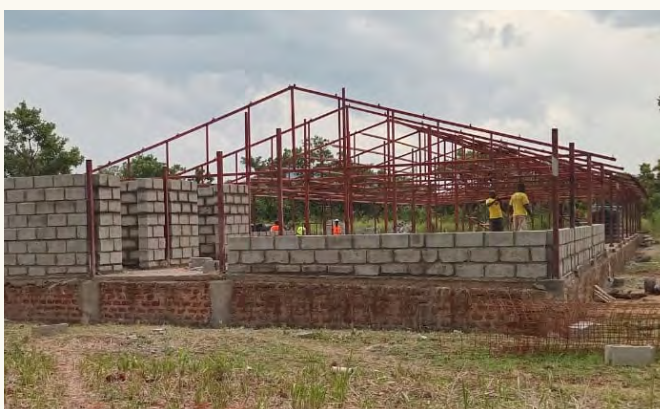
AFRUDEC pig barn under construction
