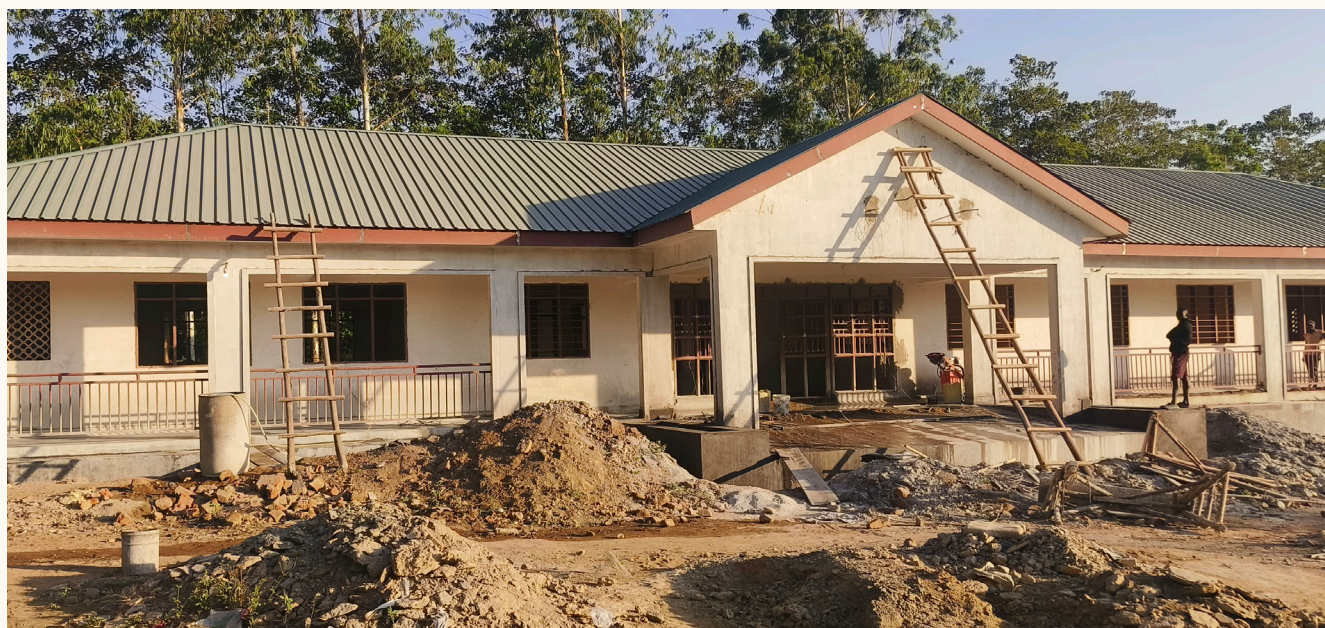
Providence Medical Center under construction at AFSS
