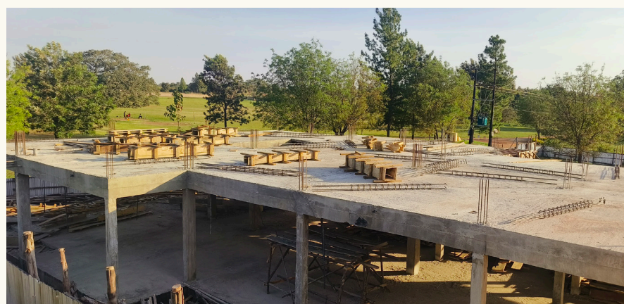
AFSS Admin Building under construction
