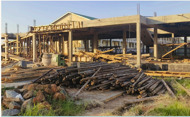
AFSS Admin Building under construction
