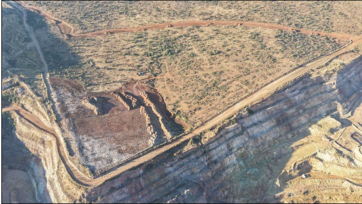
Road moved, powerline being moved and clearing in progress in late November
