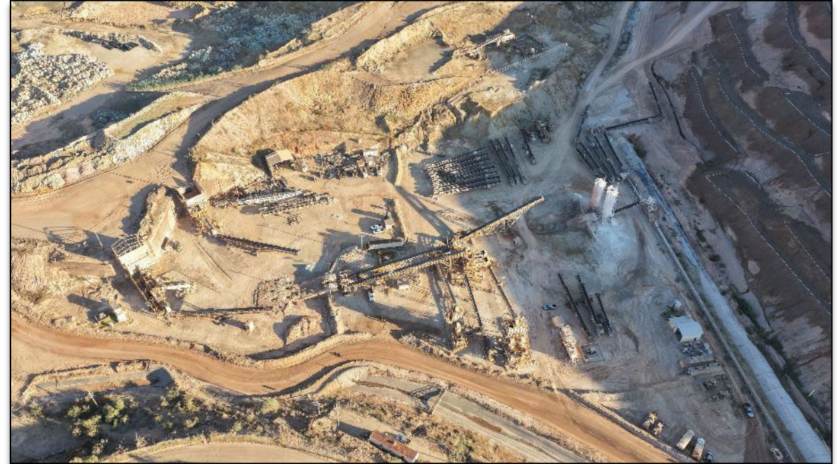
Restart maintenance on crushing circuit at 70% completion prior to restart in December
