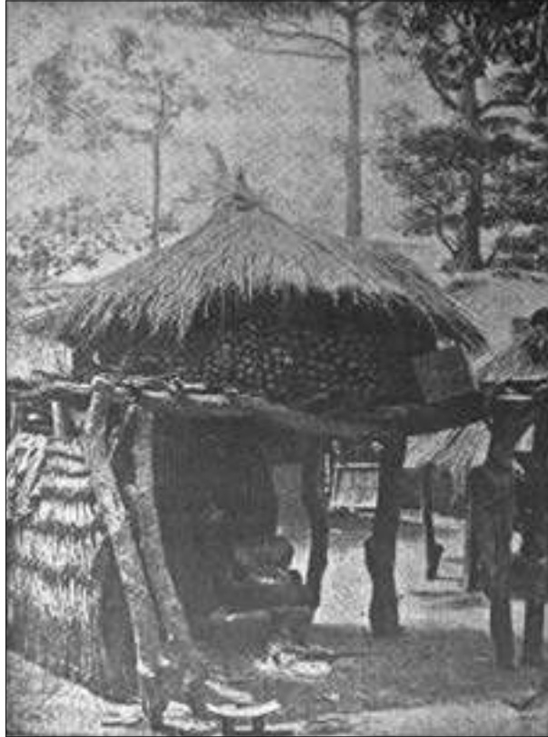
Maize Granary, Under it a hearth for the smoking of corn, to dry it and to protect it against maize beetles
