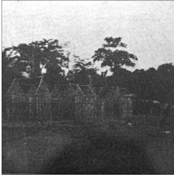
Negro Huts under Construction
