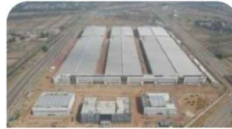
Over 125,000 sq. m. PEB installation for a multinational home appliance manufacturer based out of Noida
