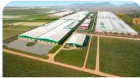
Over 285,000 sq. m. PEB installation for a textile plant for a major textile company at Hoshangabad, Madhya Pradesh
