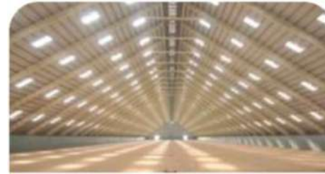
Approx 90,000 sq. m. 'A' frame structure with a centre height of 42 metres and clean span of 84 metres specially designed for the sugar storage requirements for a major Indian sugar company in Kandla, Gujarat
