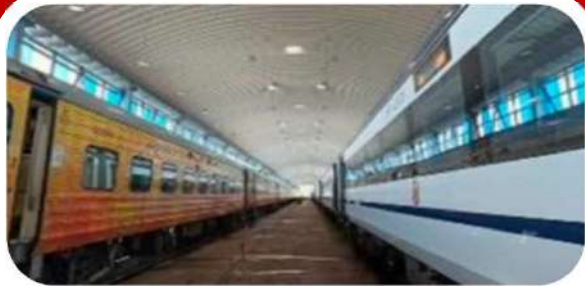
Vande Bharat Mumbai Central Pit Line Shed
