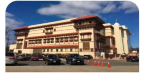
Over 18,000 sq. m. PEB installation for a temple at New Jersey, US
