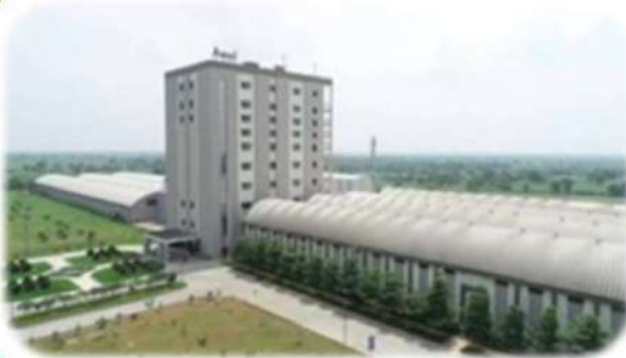
Self-supported roofing structure for a major Indian milk co-operative society at Anand Gujarat
