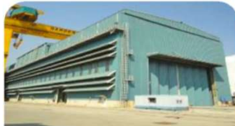
Approx 3,000 sq. m. PEB installation with a retractable (openable) roof structure for a Kolkata based shipyard
