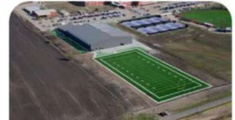
Over 5,500 sq. m. PEB installation for an indoor multi-use facility at Texas, US
