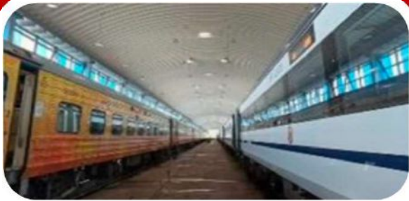
Vande Bharat Mumbai Central Pit Line Shed
