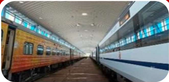
Vande Bharat Mumbai Central Pit Line Shed
