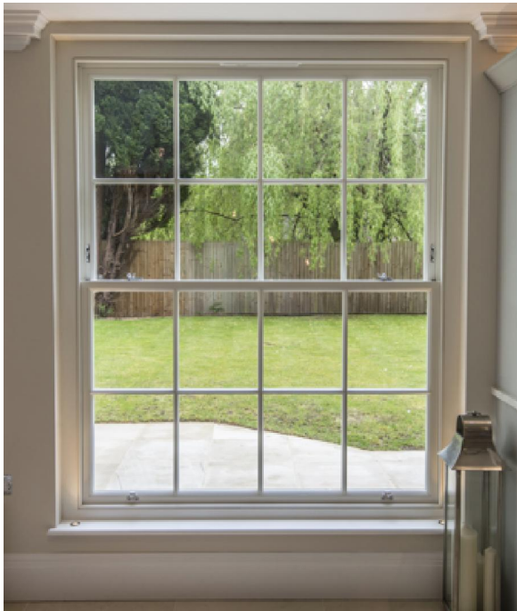
FINAL STAGE: WINDOWS ON SITE
