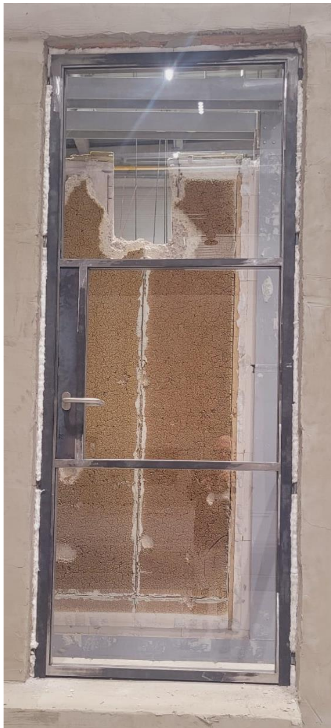
Photo. 3. Door No. II examined from the inside.
