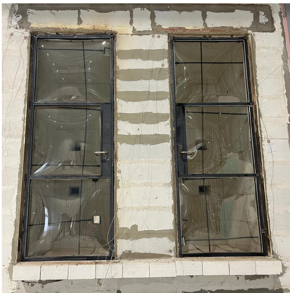
Photo. 4. Removal of the test element after the end of the test (36 min).
