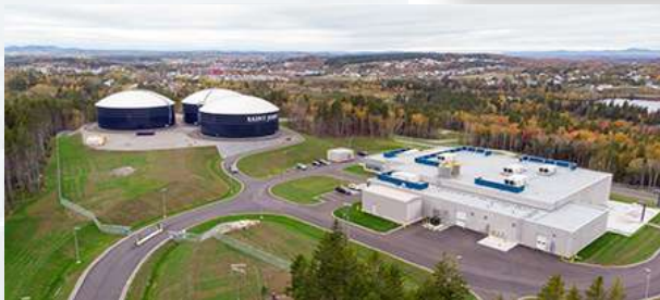
Loch Lomond Water treatment plant – St John, NB, Canada
