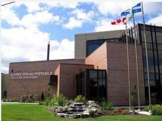
Water treatment plant of Ste Marie de Beauce, Canada
