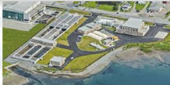
Eastern passage wastewater treatment plant – Halifax, Canada
