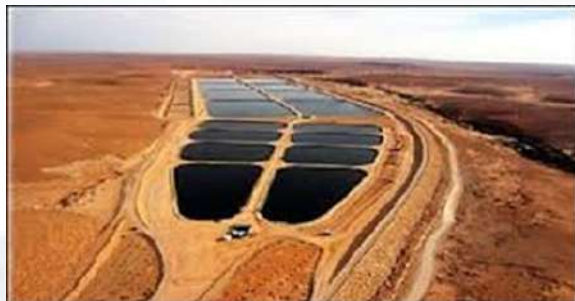
Wastewater treatment and flood protection in the M'Zab Valley, Ghardaia wastewater Treatment Plant, Algeria
