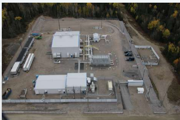
Natural gas compression stations construction management, St Maurice, Quebec, Canada - 80M$
