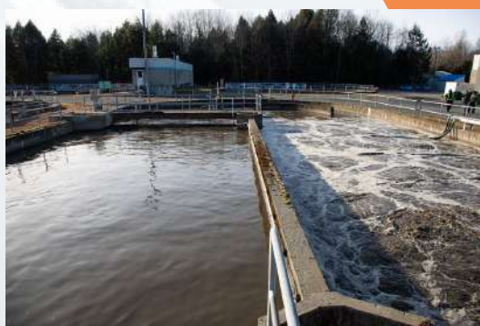
Wastewater treatment plant upgrades, Cowansville, Quebec, Canada
