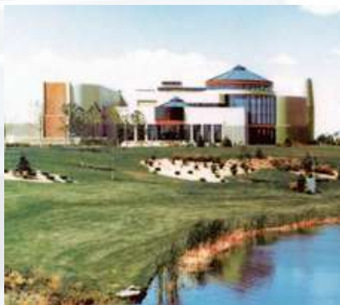
Construction management and commissioning, South Shore Wastewater Treatment Plant and Sewerage Network (CERS), Longueuil, Quebec, Canada - 330,000 m 3 /day
