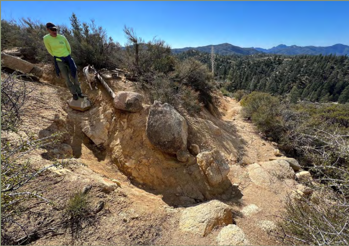
Before: A deeply channelized switchback with major erosive damage from water flowing through the corner.
