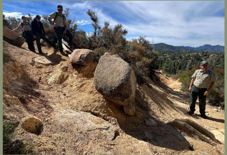
After: The corner is armored with rocks and the deep channel is filled with durable materials. New drains installed above the corner will slow future erosion.
