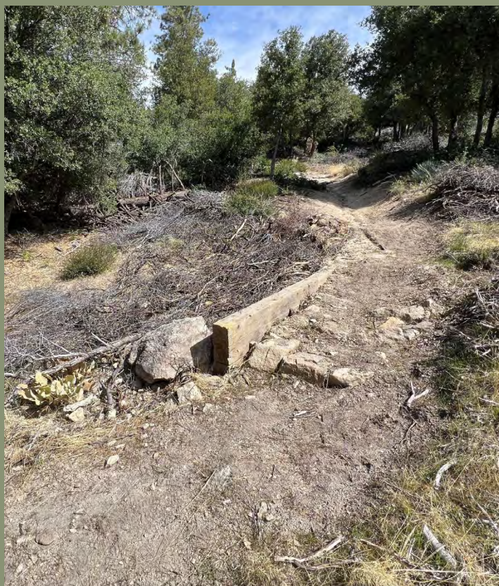
After: Steps are deconstructed and the trail is shifted out of the drainage path. The tread is armored with local rock, and the corridor is narrowed with vegetation.
