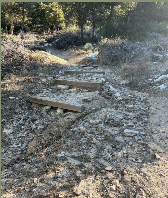
Before: Wooden steps are directly in drainage, and water erosion is causing users to avoid using the steps, widening the trail corridor.
