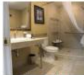
Curbless shower & roll-under sink
