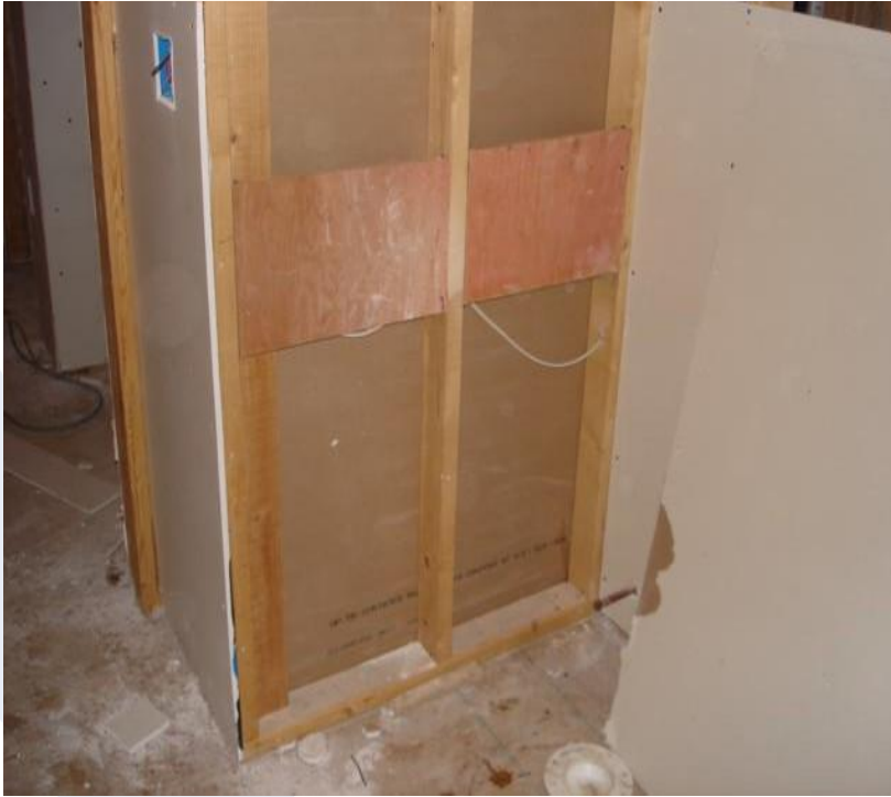
Wall reinforcements in shower and around toilet; potentially in hallway
