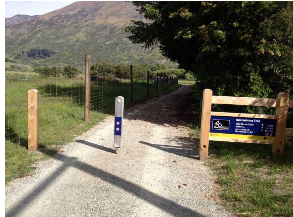
Figure 21. Image showing removeable bollard with luminous and reflective signage.
