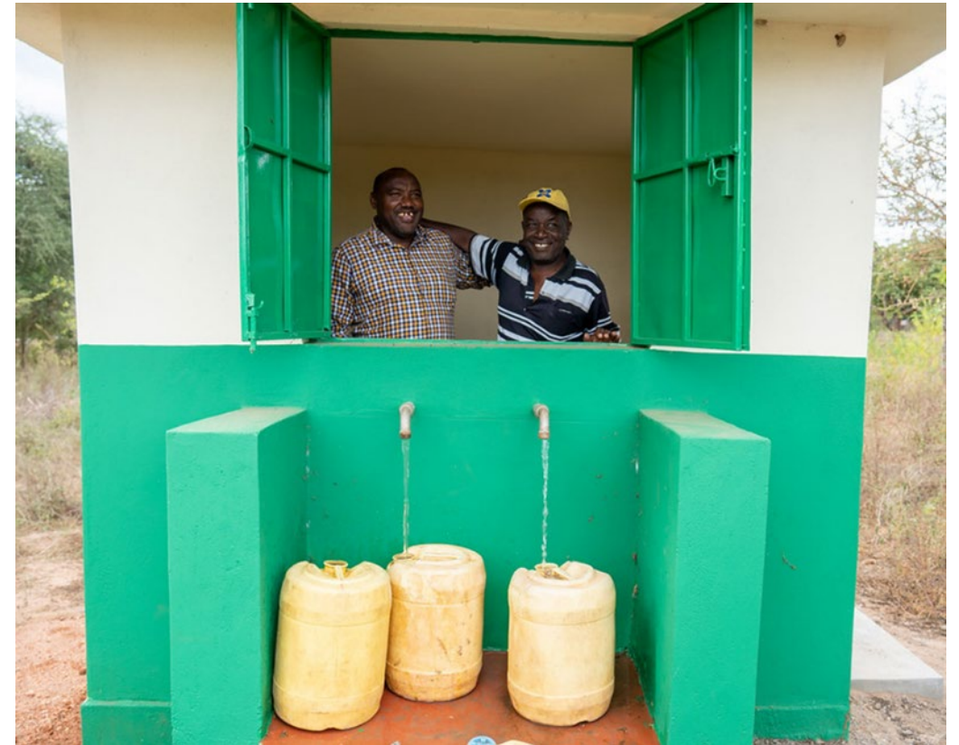
A community water kiosk at Itaava Market, which serves over 1,500 residents with reliable access to clean water.
